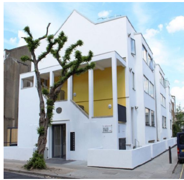
Artic Street, Housing Coop, Camden
