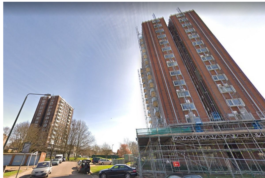
Many London local authorities have to invest in building safety improvements for their own stock (Picture above: the Granville Road tower blocks in Childs Hill during recladding, Source: Google)
