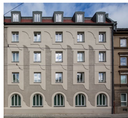
Munich. Housing block renovation.
